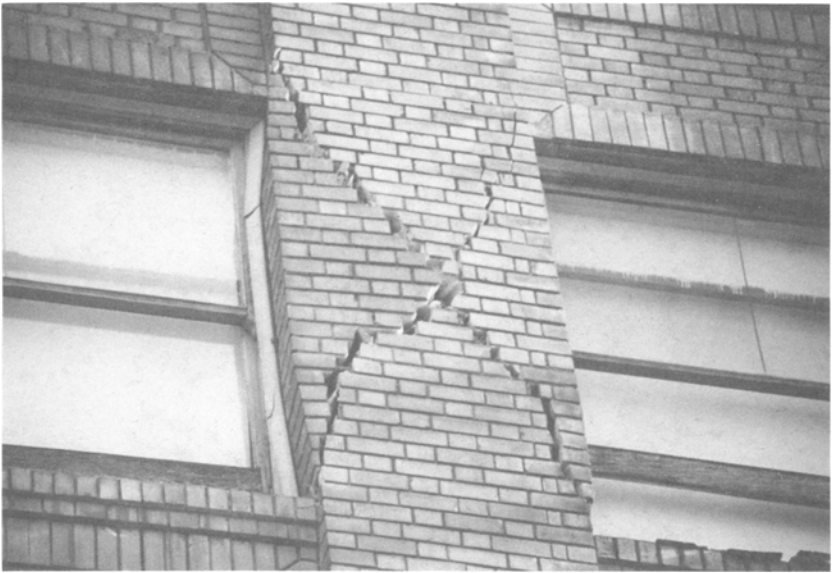
FIG. 4. In-Plane Shear Failure of URM Pier (Oakland, Loma Prieta Earthquake)
