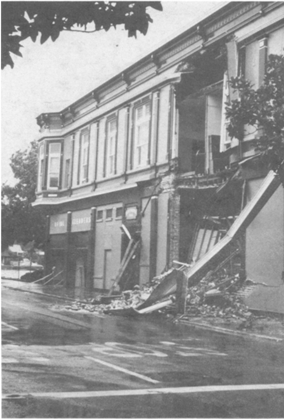
FIG. 7. Out-of-Plane Failure of URM Wall at Center of Building due to Excessive Diaphragm Flexibility (Santa Cruz, Loma Prieta Earthquake)
