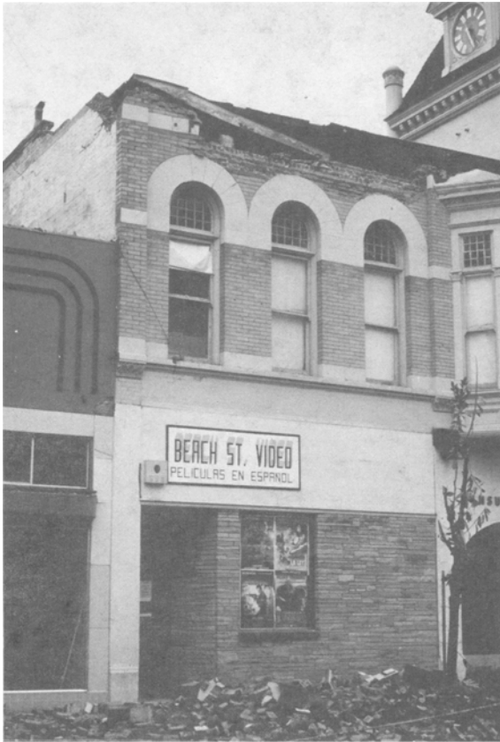
FIG. 8. Parapet Failure of 100 Front Street Building (Watsonville, Loma Prieta Earthquake)
