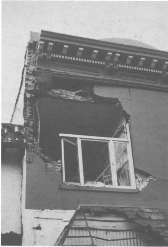
FIG. 12. Combined out-of-Plane/in-Plane/Pounding Failure (Santa Cruz, Loma Prieta Earthquake)
