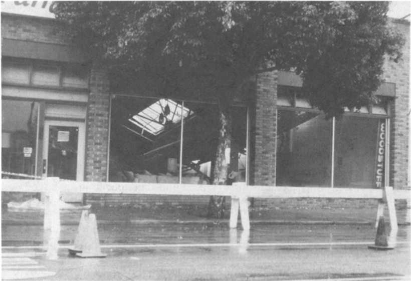
FIG. 1. Typical Failure due to Slip of Roof Joists off Their Wall Supports (Santa Cruz, Loma Prieta Earthquake)
