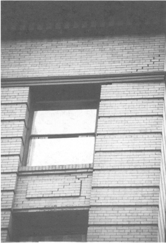
FIG. 3. In-Plane Shear Failure of URM Spandrel Beam (San Francisco, Loma Prieta Earthquake)
