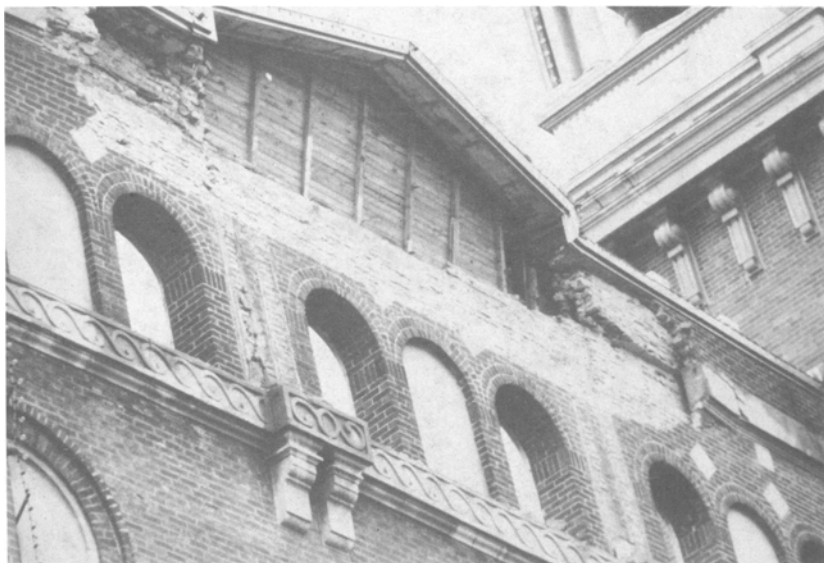
FIG. 10. Failure due to Combined out-of-Plane Failure of Parapet and Inadequacy of Collar Joint in Multiwythes URM Wall (Quebec City, Saguenay Earthquake)
