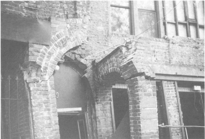
FIG. 5. Flexural Failure of Slender URM Column (Los Gatos, Loma Prieta Earthquake)
